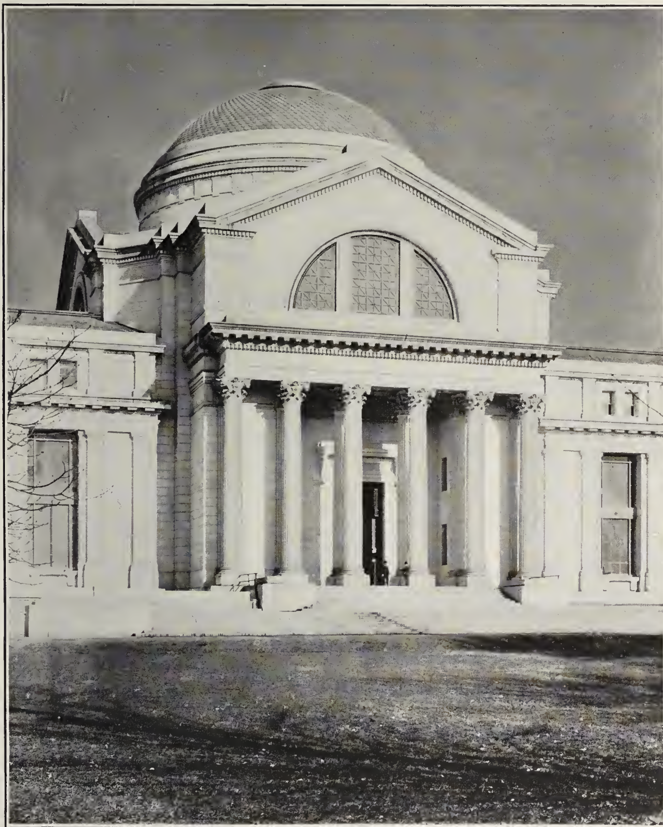
SOUTH PAVILION, ROTUNDA, PORTICO AND APPROACH.
